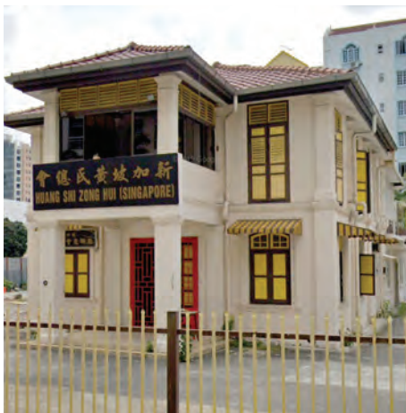
Former Huang Clan Singapore Association building at 16, Lorong 35 Geylang.
