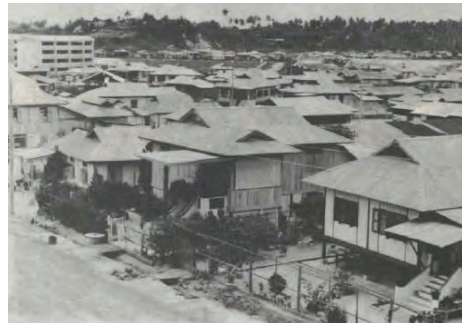
Bungalow-type houses of the Malay Settlement at Jalan Eunos.
