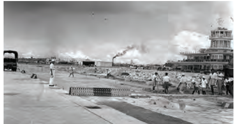
Indian labourers at work on the runway at the Kallang Airport, 1950.
