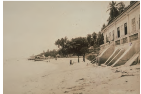
Seaside villas along Tanjong Katong. The Foreshores Act required seaside houses be built at least 15 metres from the shoreline.
