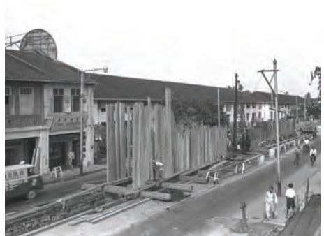
Drainage and sewerage works in progress at Geylang Road in July 1963.
