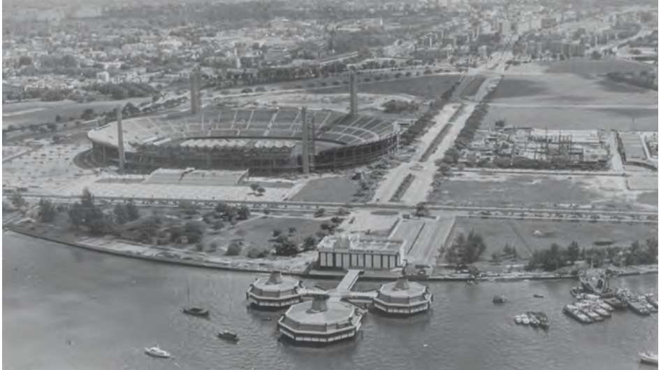
Aerial view of the National Stadium.
