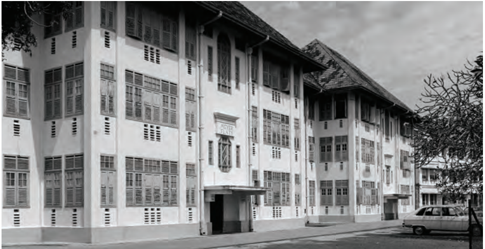
Three-storey Meyer Apartments built in 1928, taken in 1982.
